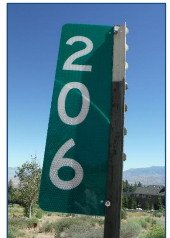
An approved reflective address marker with 4-inch numerals mounted on a fire-resistant post.
