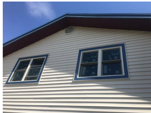
Enclosed eaves/secure vents
