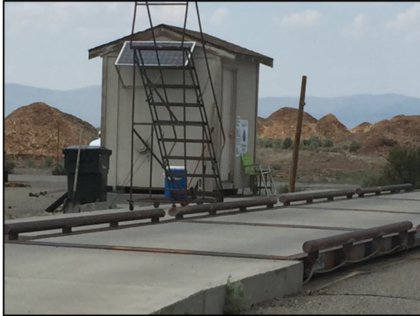
Figure 12. Pumice Valley Facility Area
