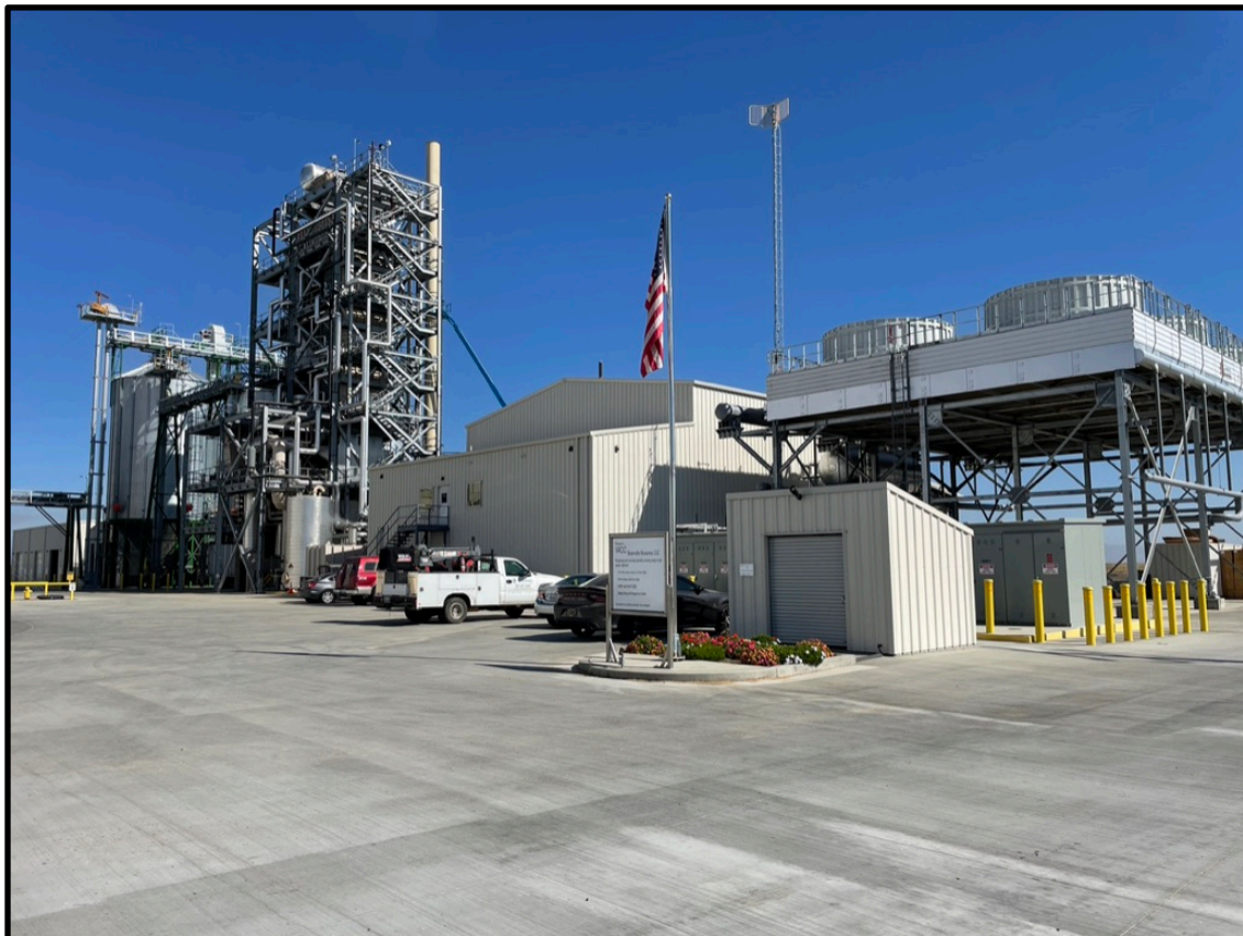
Three megawatt biomass power plant in Williams, CA
